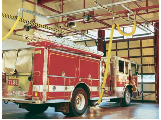
SBT emergency extraction system
